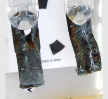
Figure 13. Electrical Conduit Strap, Day 560, Salt Water.
